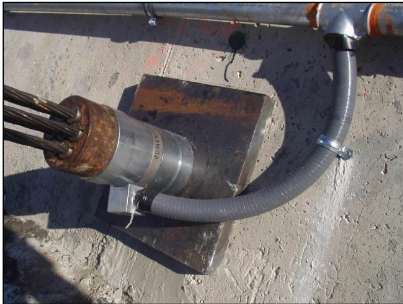
Figure 6: Bearing plate fabricated and placed between wall and loadcell distribution plate
